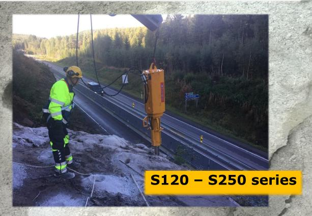
**SplitStone** -wedge technology is based on a splitting method developed in collaboration with specialized quarry companies.
